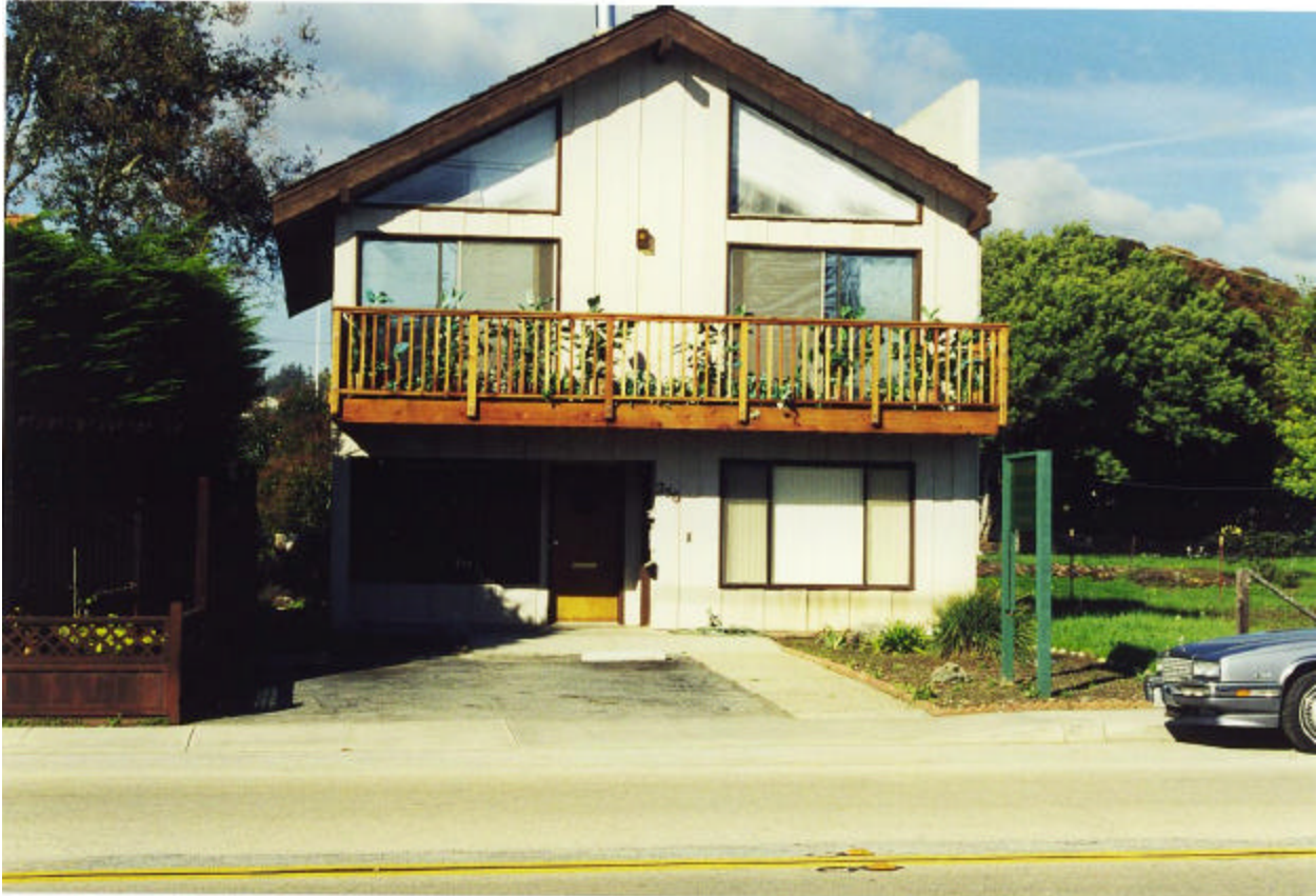
Figure 18: Office and Residential Use
