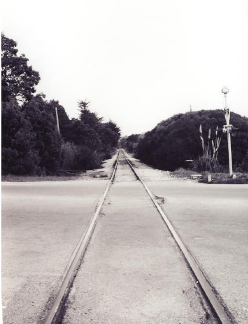
Figure 25: Existing Railroad Tracks.
