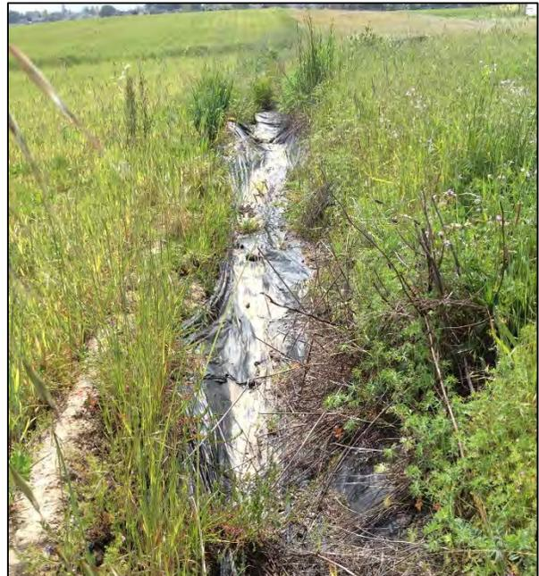
Photograph 14. View of black plastic-lined ditch along northeastern Project boundary. Ditch drains southwest.
