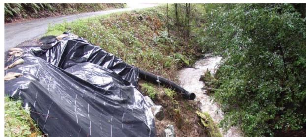
THIS ROAD SLIP OUT DELIVERS SEDIMENTS DIRECTLY TO THE STREAM
