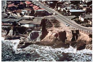
Photo 6-14. Example of outflanking. (Source: G. Griggs)
