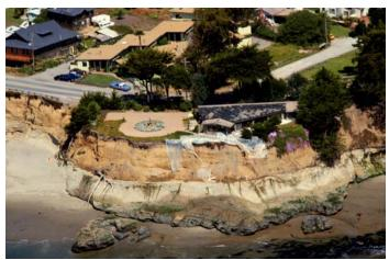
Photo 6-4. Example of bluff erosion. (Source: G. Griggs)
