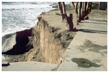
Photo 6-13. Result of wave overtopping. (Source: G. Griggs)
