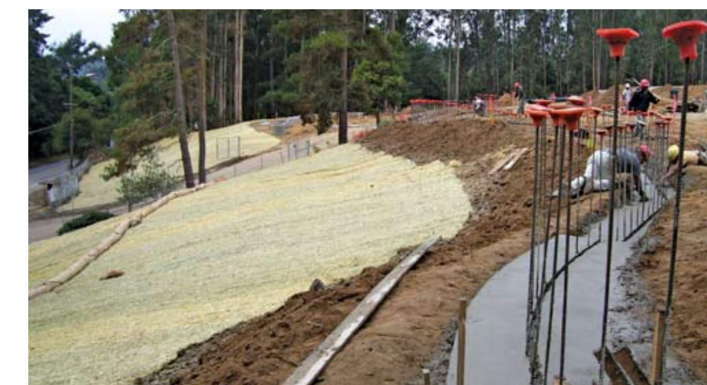
EROSION CONTROL METHODS INCLUDE BLANKETS, WATTLES (ROLLS), MULCHING AND SEEDING
