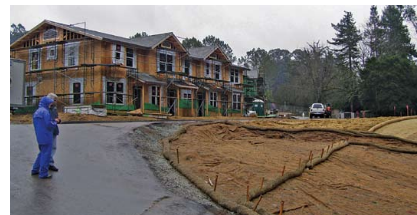
EROSION CONTROL MEASURES WORK BEST WHEN INSTALLED PRIOR TO THE RAINY SEASON
