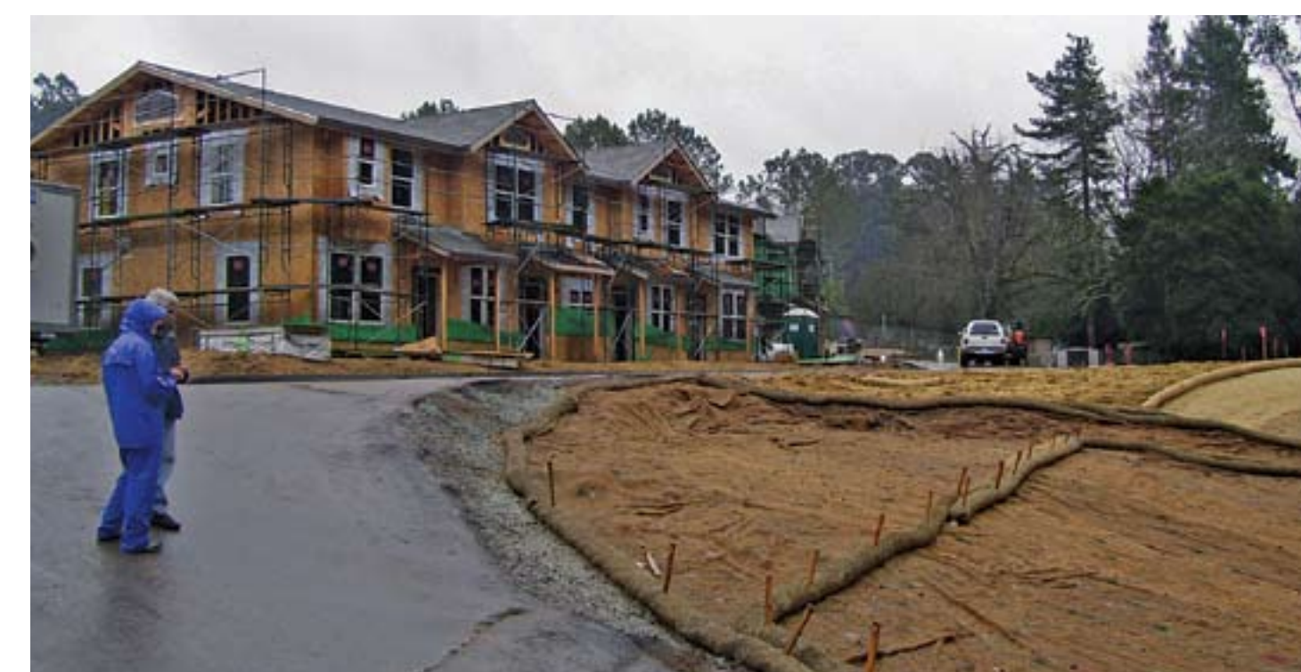
EROSION CONTROL MEASURES WORK BEST WHEN INSTALLED PRIOR TO THE RAINY SEASON
