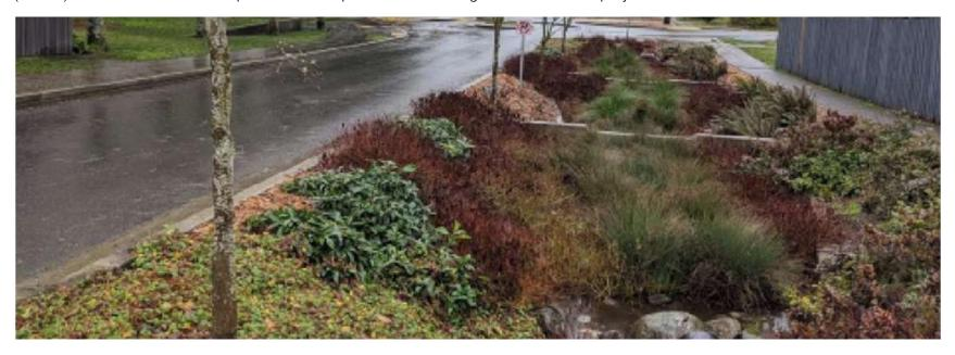
Bioswale collects and filters stormwater Photo Credit: MIG, Inc.
