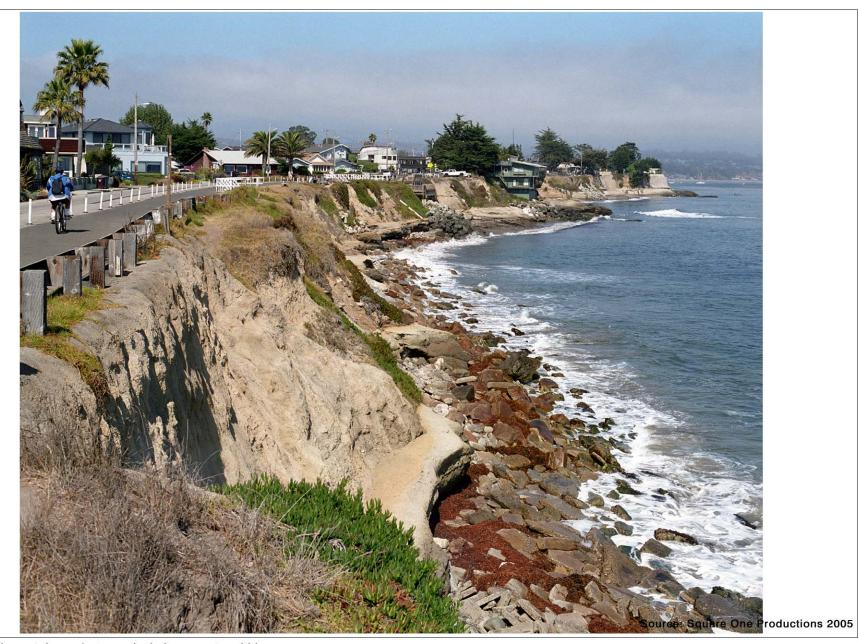
Existing conditions at the project area include concrete rubble, sculpted and colored soil nail walls constructed as emergency repairs in 2004 (lower left-hand corner of picture), white protective railing around areas of failed roadway, nonnative vegetation and minimal beach area due to the concrete rubble and rock riprap.
